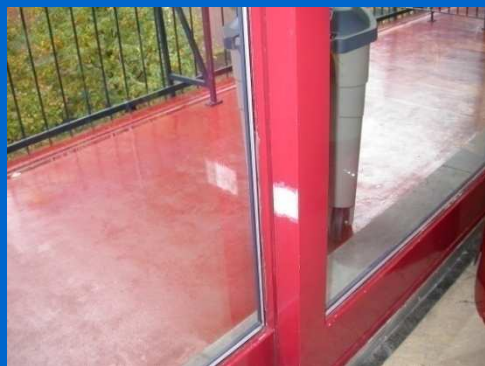
Painting containing lead but not representing an immediate risk (inaccessible or smooth surface)
