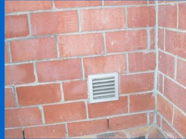
From the outside, the size of the air inlet is barely 20 cm sur 20 cm
