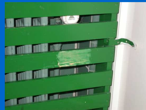
Painting containing lead but not representing an immediate risk (inaccessible or smooth surface)
