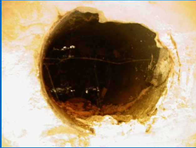
From inside, the air entrance is not clear !
